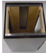
Wood Mounting Frame & Duct Cover—TOP VIEW
